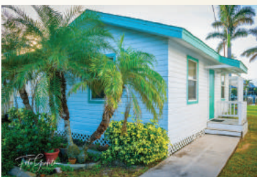
Newly renovated cottage.
